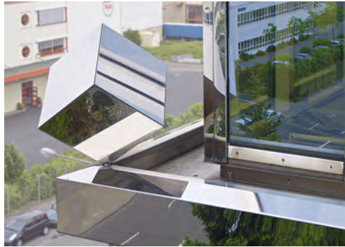
Bright annealed facade cladding before and after cleaning: Standard maintenance operations return the highly reflective surface to its original lustre. Photo: Christian Pohl GmbH, Cologne (D)
